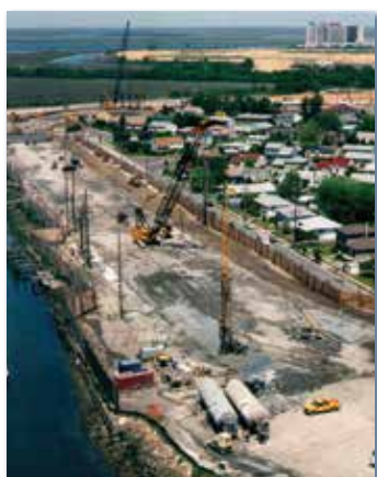
Above: Excavation support begins for construction of Atlantic City, NJ's expressway extension.
